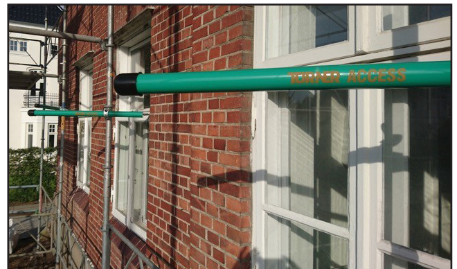
The newly developed wall anchors from Nordic Platform are made of composite and is characterized by its strength and color possibilities. Here is the scaffolding supplier Turner who has chosen his own color and printed the company name. Photo: Nordic Platform.
