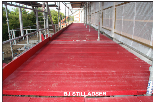
Construction site in South Denmark Photo: Nordic Platform
