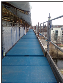
Construction site in Oslo Photo: Nordic Platform
